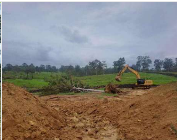
Figure 3. During Clearing Works:
