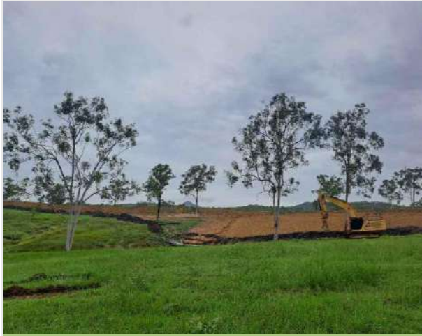
Figure 4. During Clearing Works:
