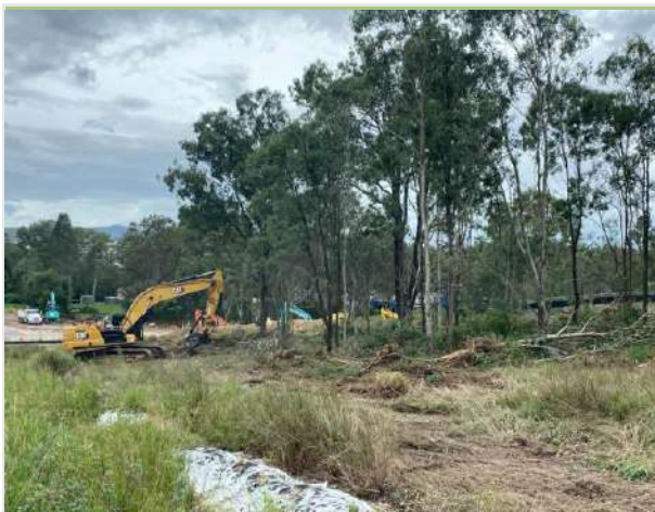
Figure 2. During Clearing Works:
